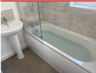
BATH FILLED & OVERFLOW TESTED ✓
